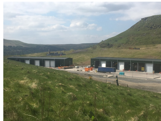
Solar PV Installation at Silent Valley Waste Transfer Station
