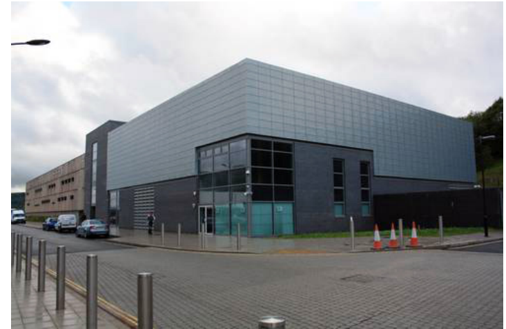
Energy Centre at 'The Works'
